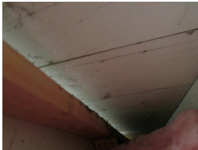
drywall stops short of roof sheathing
