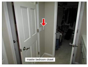
(5) There were cover plates missing at several outlets, creating shock hazards. Replace the missing cover plates.
