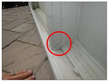
(2) The first floor patio door was starting to rot at the bottom corner of the mullion on the west side. Have this door serviced to help forestall the rotting.
