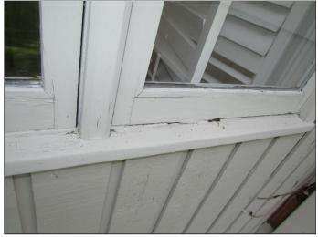
(2) The window at the back of the house indicated in the photo below was beginning to rot at the bottom corners of the mullion, and should be serviced to help forestall further deterioration.
